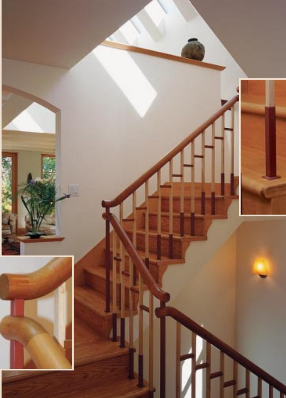
**Uncomplicated elegance.** Simple round handrails intersect with square steel tubing to form the newels, while steel-tube boots hold thin maple balusters connected with the mahogany bridges. Photo taken at F on floor plan.
